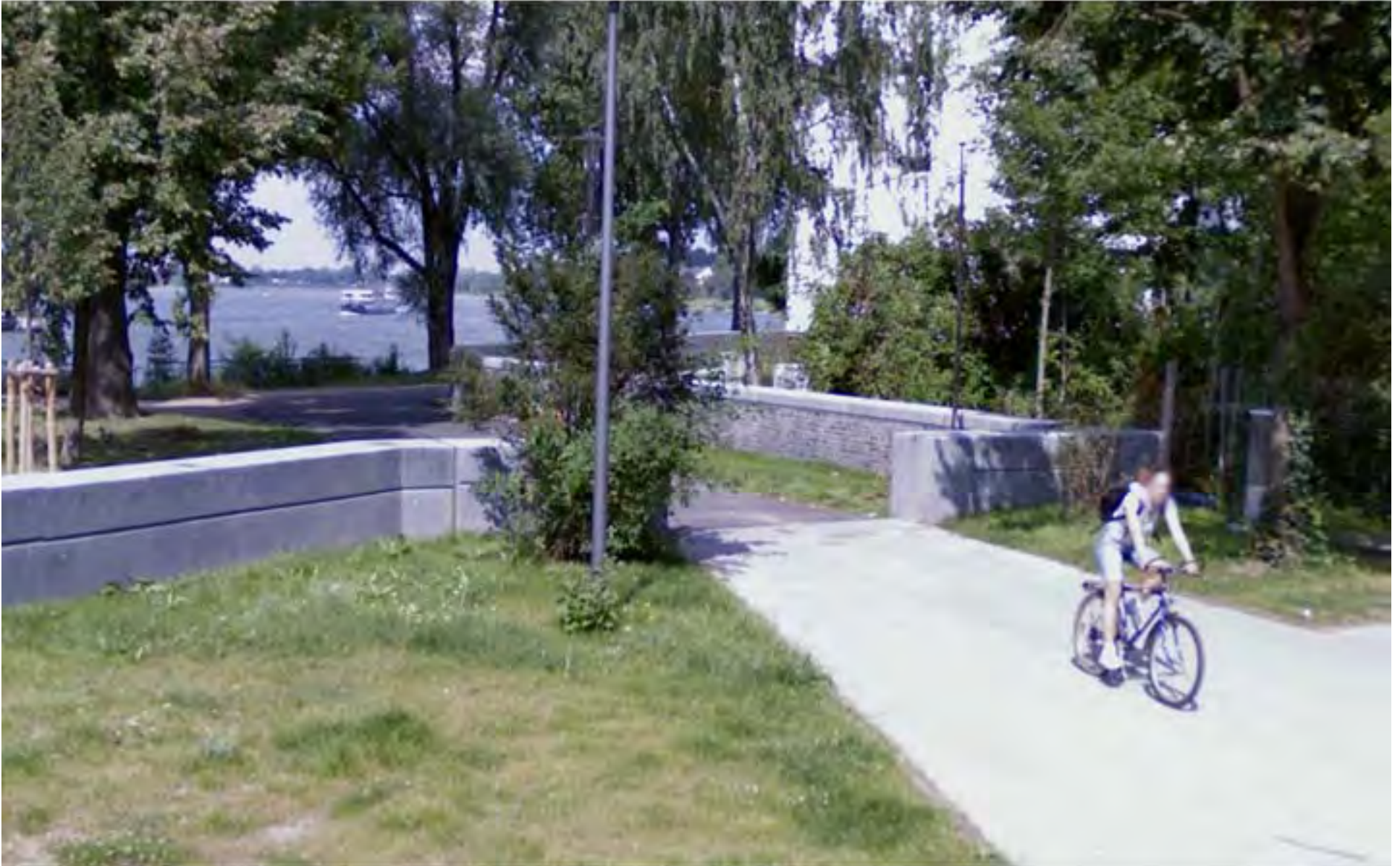
Floodwall with removable gates, Cologne, Germany.
