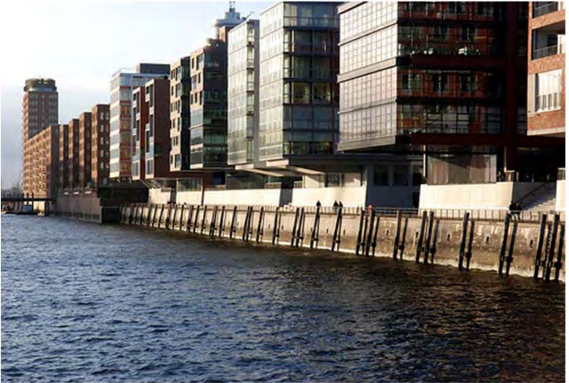
Buildings have a “hardened” 1st story along a wide pedestrian walkway.
